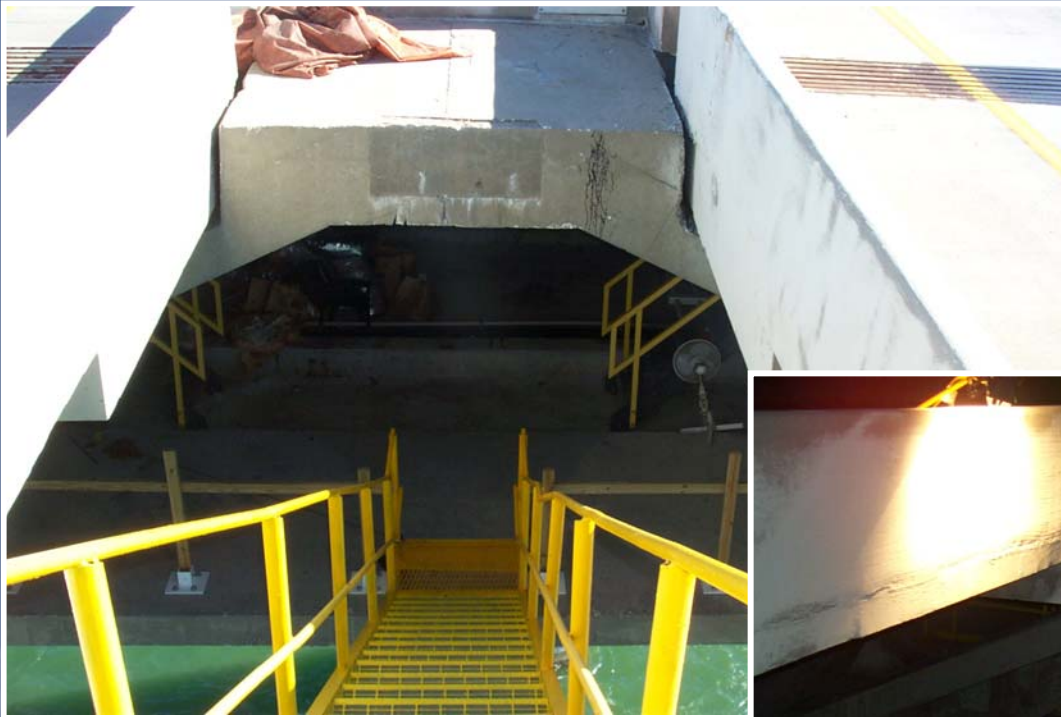
Access Stairs Segmental Transition 2003
