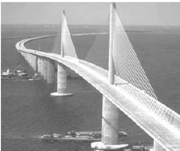
Figure 3: Oblique view clearly showing the disparity between the widths of the piers and pylons
