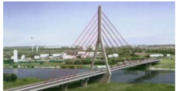
Figure 9: A-frame solution to torsion problem
