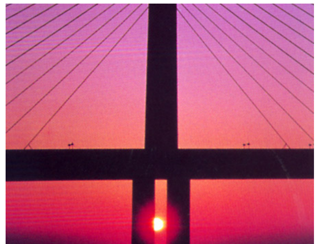
Figure 18: A clear view of the use of twin slender piers to add flexibility.
