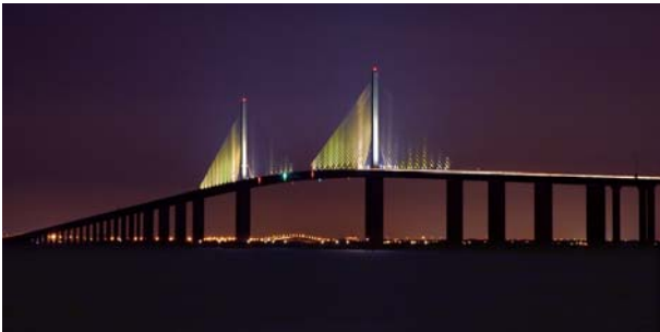
Figure 4: The Bridge at night.
