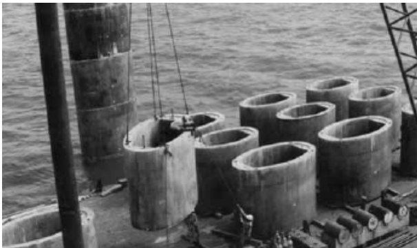
Figure 11: Concrete segments on large cranes had to be used into position.
