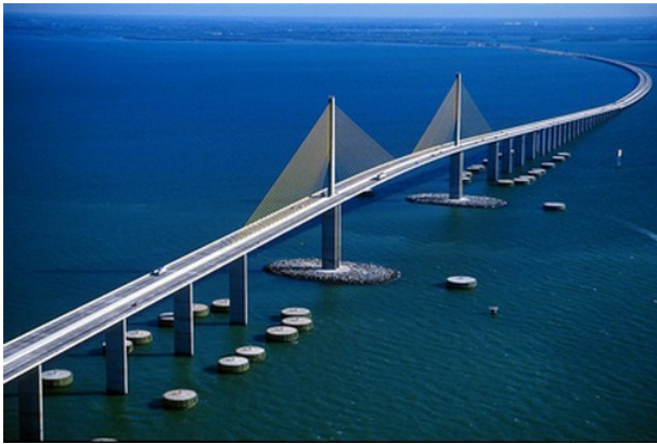
Figure 10: View of the protective concrete dolphins surrounding the bridge.
