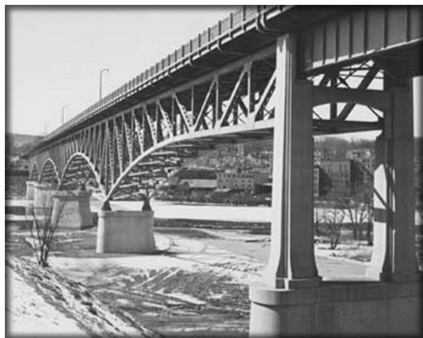
Figure 1 The Memorial Bridge in Augusta, Maine.
